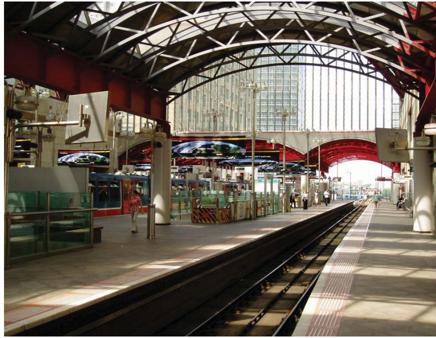
A light rail station at Canary Wharf in London, UK sits between two office towers and links several transit lines under a light and airy atrium.
